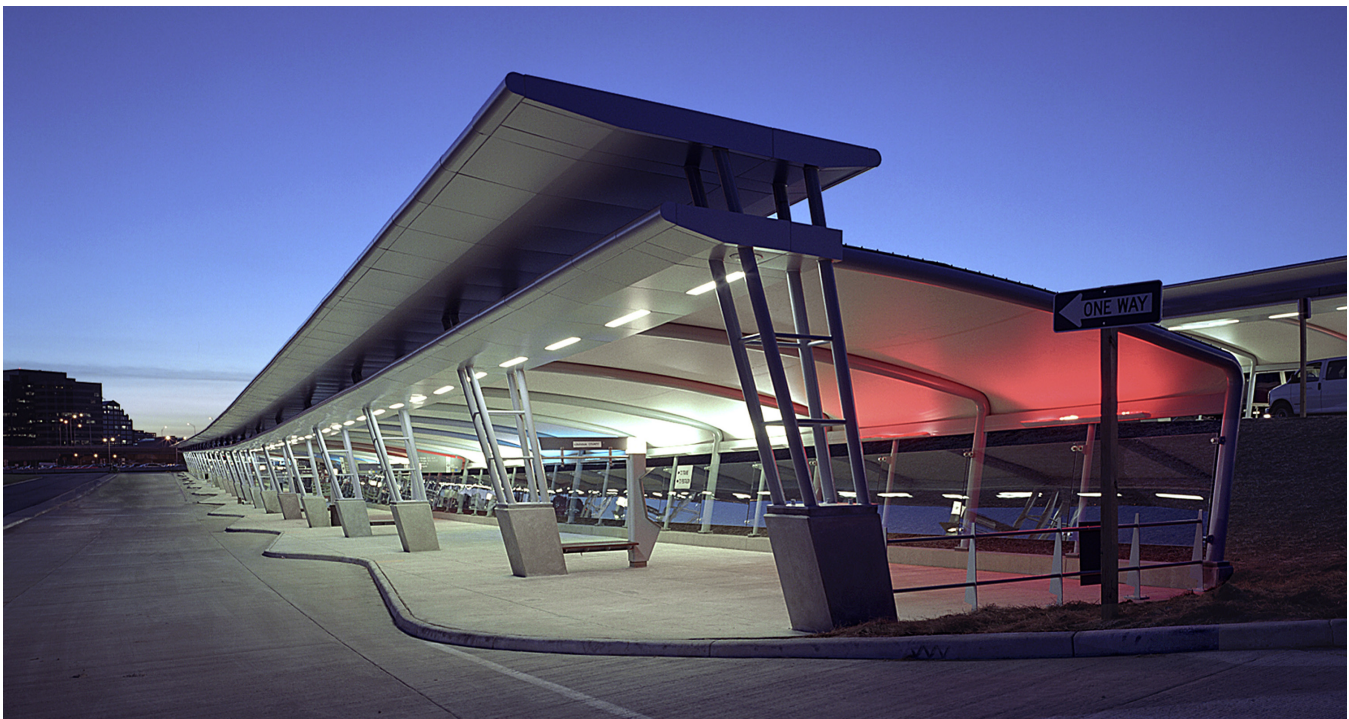
Figure 30. Bus loading/unloading area of the Pentagon Metro Entrance Facility. Photo by Sisson Studios, Inc, courtesy of HDR Architects.
