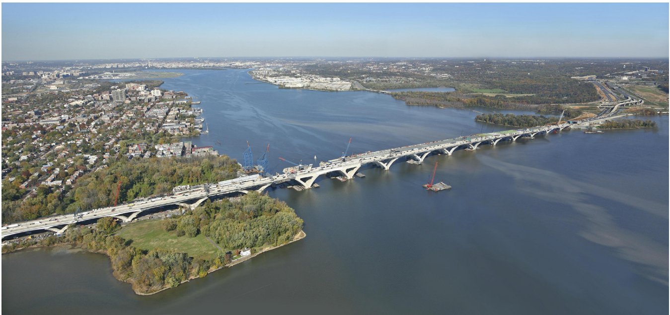
Figure 34. Aerial view looking north at the Woodrow Wilson Bridge. Photo by Top Shots photography, courtesy Potomac Crossing Consultants.
