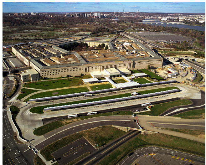
Figure 31. Aerial image of the Pentagon Metro Entrance Facility. Photo by Sisson Studios, Inc. courtesy of HDR Architects.
