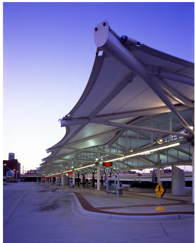
Figure 2. Canopy of The Rapid, Surface Transportation Center. Photo by Chuck Heiney, courtesy of Progressive AE.
