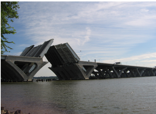
Figure 35. View looking at the Woodrow Wilson Bridge opening. Photo by Potomac Crossing Consultants.
