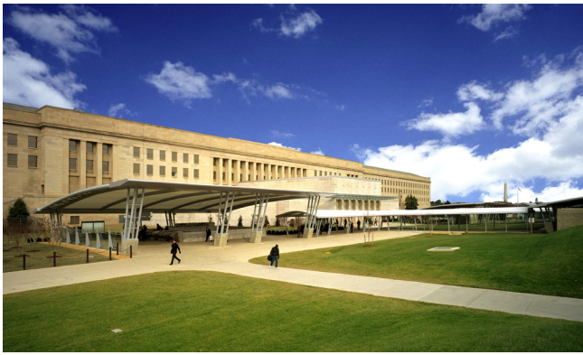
Figure 32. Pedestrian entrance of the Pentagon Metro Entrance Facility. Photo by Sisson Studios, Inc, courtesy of HDR Architects.
