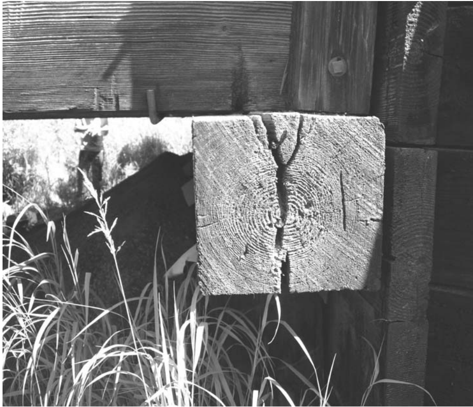
Illustration 2.1: The effect of downward deflections on span end support structures.
