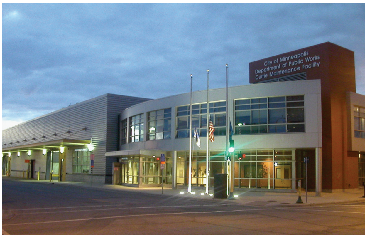
5.4 Currie Street Maintenance Facility main entrance.
