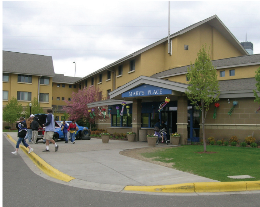
15.4 Mary's Place is a transitional housing facility that prepares residents for independent living.
