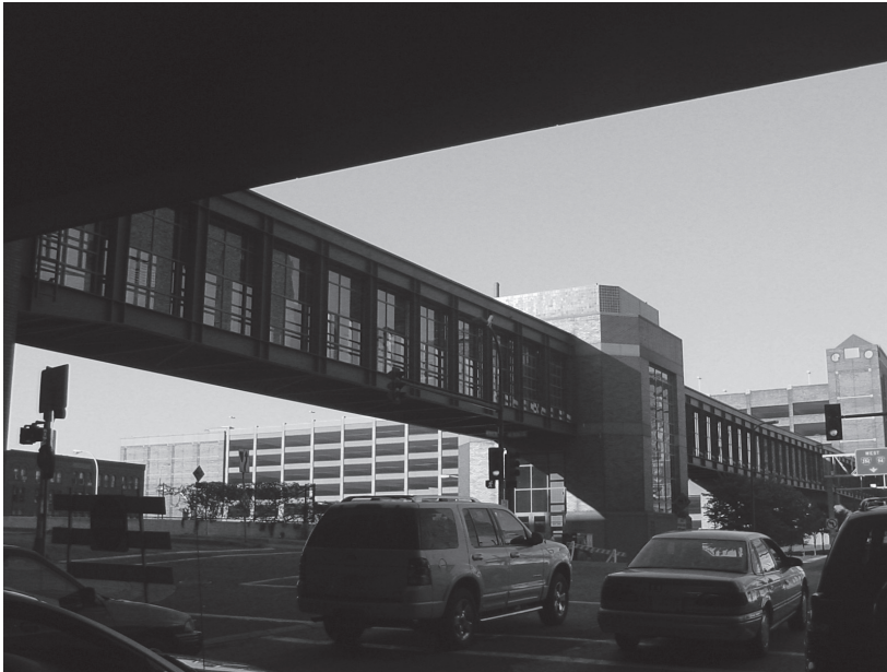
8.2 Skyways connect to the garages creating a physical divide.
