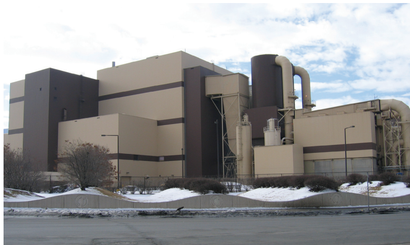
5.3 Exterior view of gas scrubber and fly ash bagging system.
