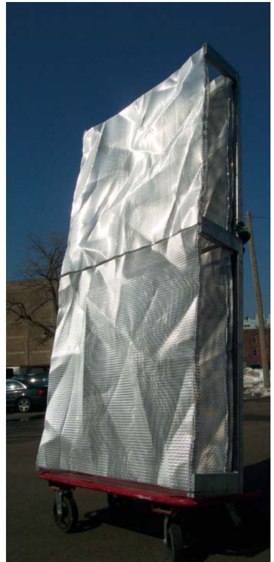
7.6. Right. A sample of the final aluminum panels and the steel structure that holds them away from the weather wall.
