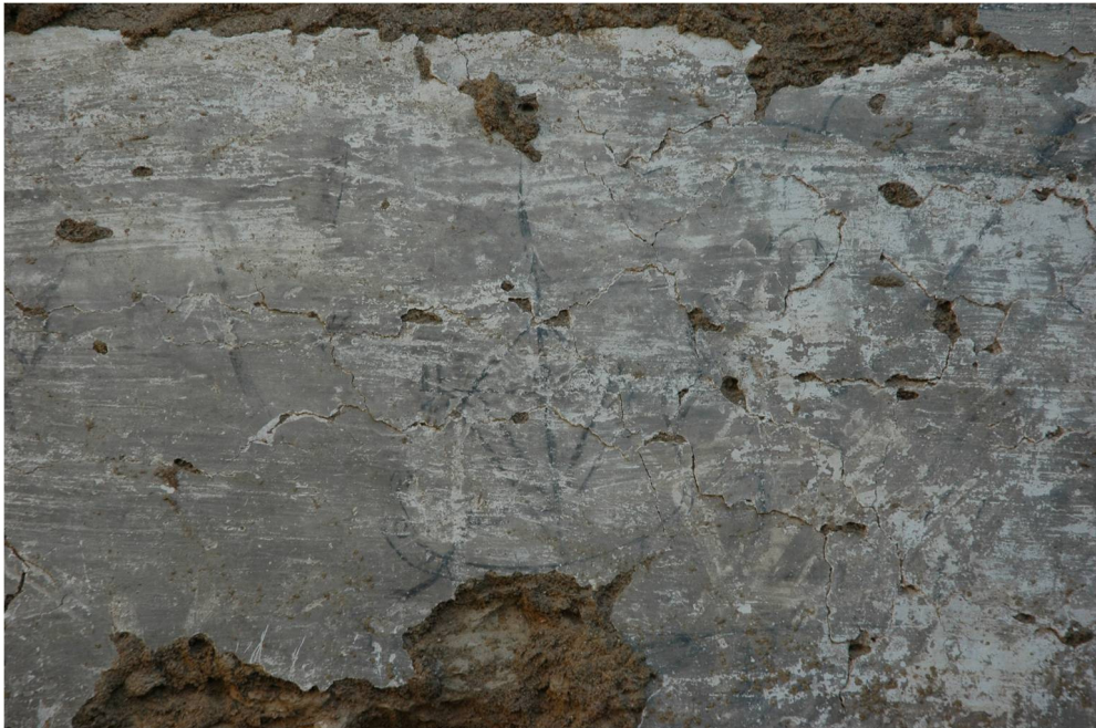
Plate 53: detail of graffiti on the north wall of room B6.
