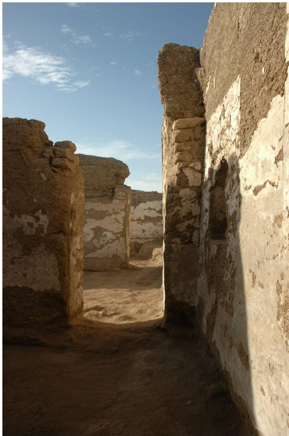
Plate 51: view of the passageway from room B6 to rooms A46 and B5 (to S).
