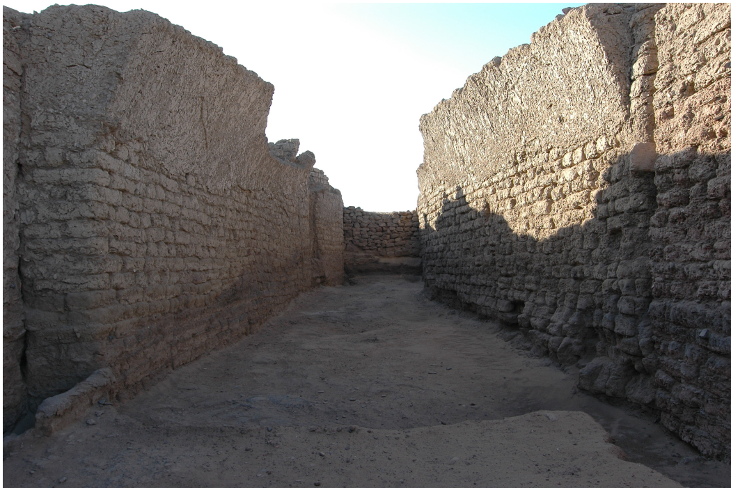
Plate 69: view of passageway B11 (to W).
