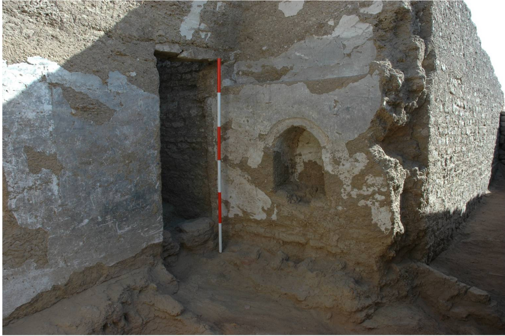
Plate 56: view of the northeast corner of room B6 (with door leading to staircase B8).
