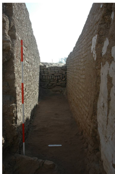
Plate 59: view of corridor B7 (to E).
