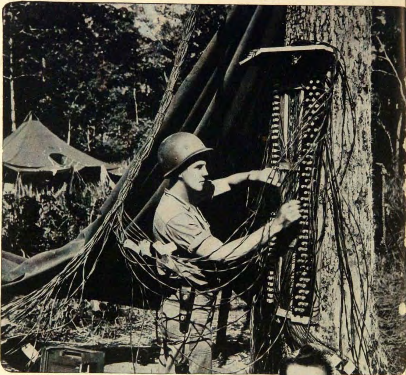
U. S. Marine setting up a telephone switchboard on an island "somewhere in the Pacific"
