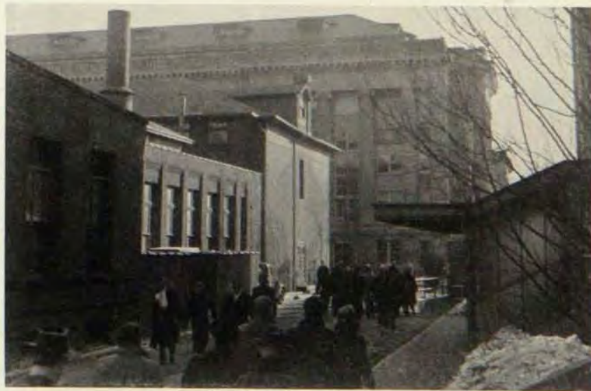
The present Mechanical Engineering building is a combination of two buildings, one constructed in 1900 and the other in 1901. In 1926 the space between the two was covered over to make the present rambling structure. The interior construction is wood and the rooms are poorly lighted and poorly ventilated. In many places, special props have been inserted under the floors to carry the weight of the heavy machines at which students work.
