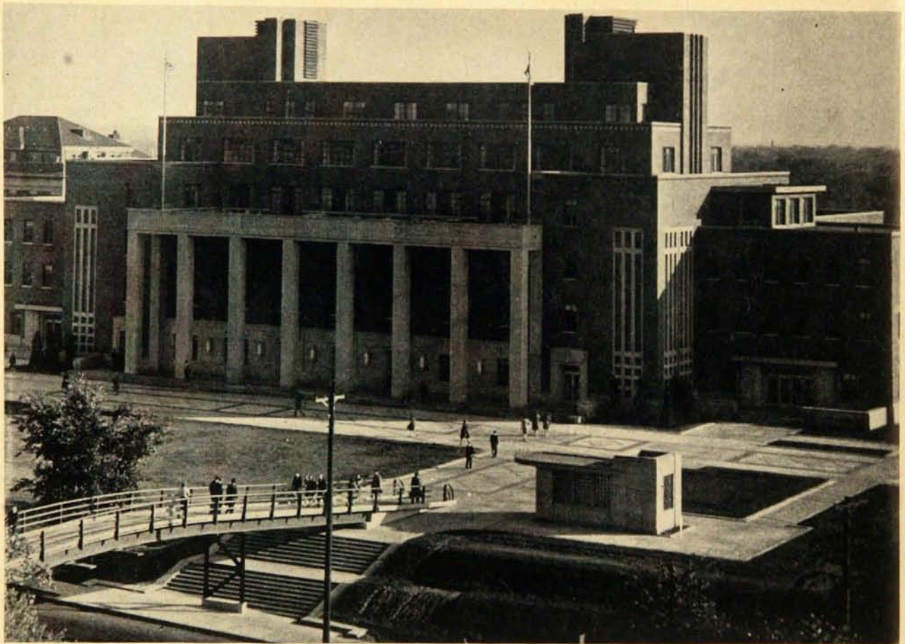
View of Coffman Memorial Union showing one of the two pedestrian bridges across Washington Ave.
