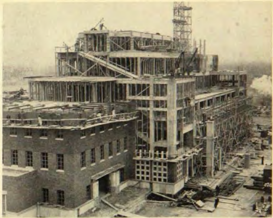
Work is progressing rapidly on the construction of Coffman Memorial Union
