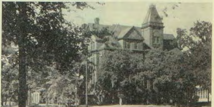
Men may come and men may go but this veteran campus building continues to serve the university as the home of the School of Business Administration.
