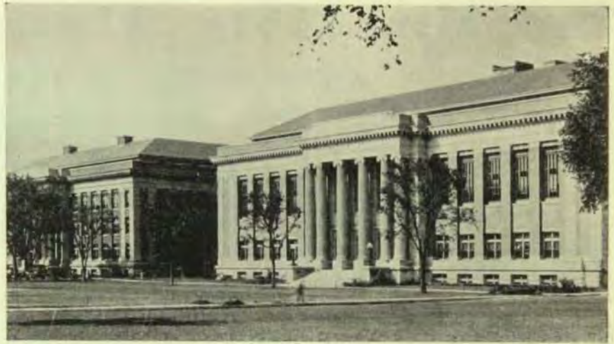
Chemistry Building and Library on the Mall
