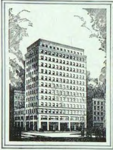
Home Office Building
