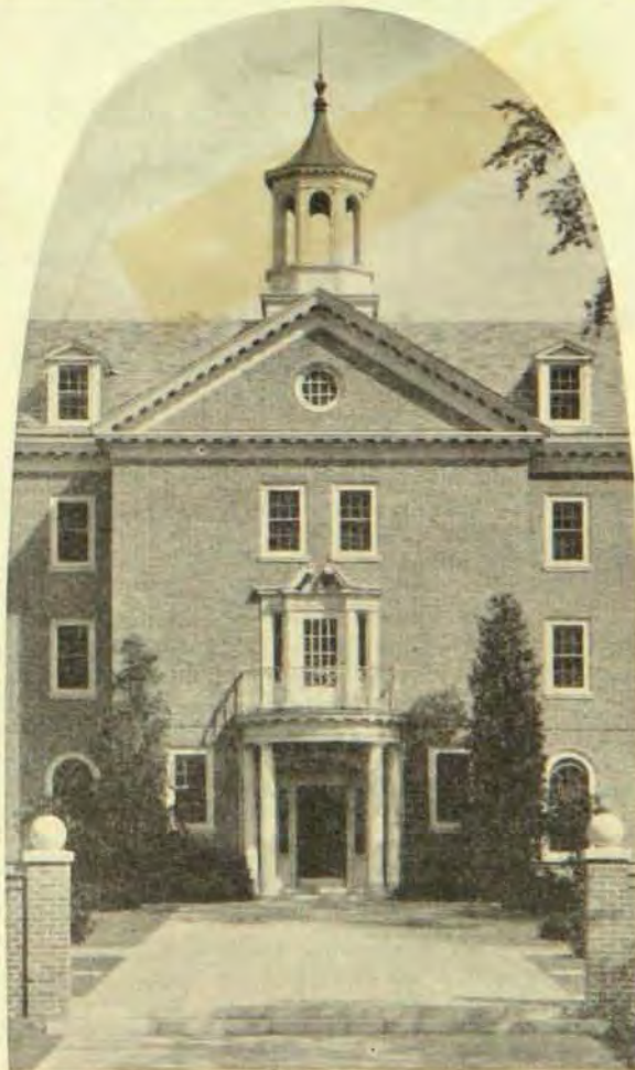
Entrance to Pioneer Hall
