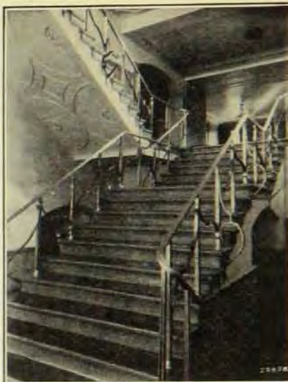
New Stairway in the Minnesota Union
