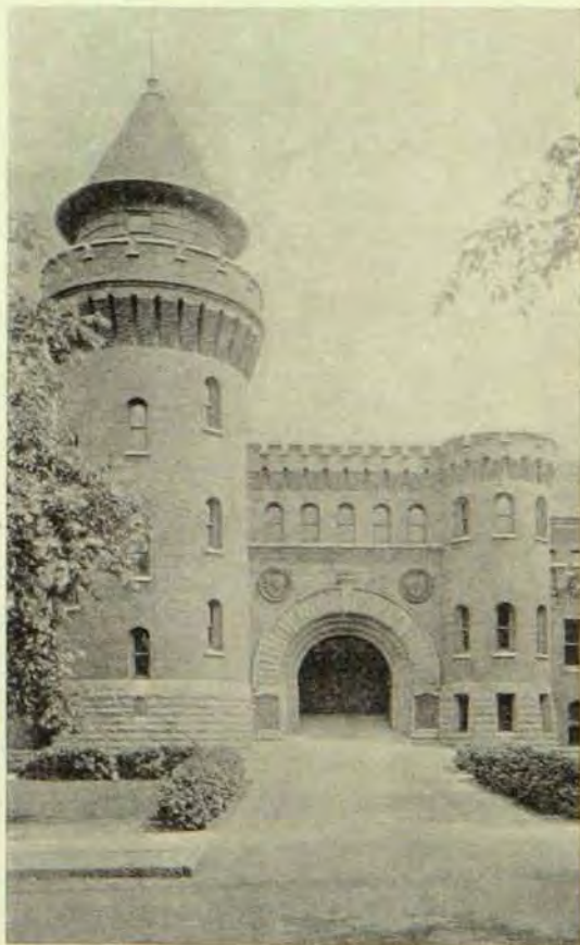
ENTRANCE TO ARMORY
