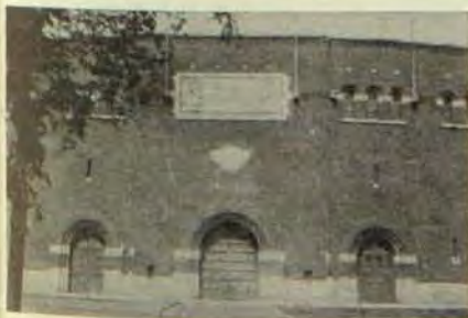
MEMORIAL STADIUM GATE
