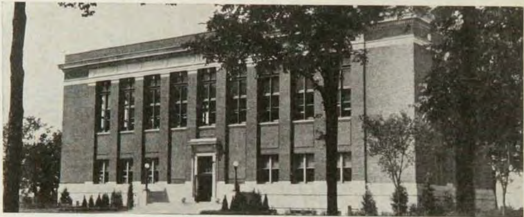
New Law School Building between Mines and Pharmacy Buildings
