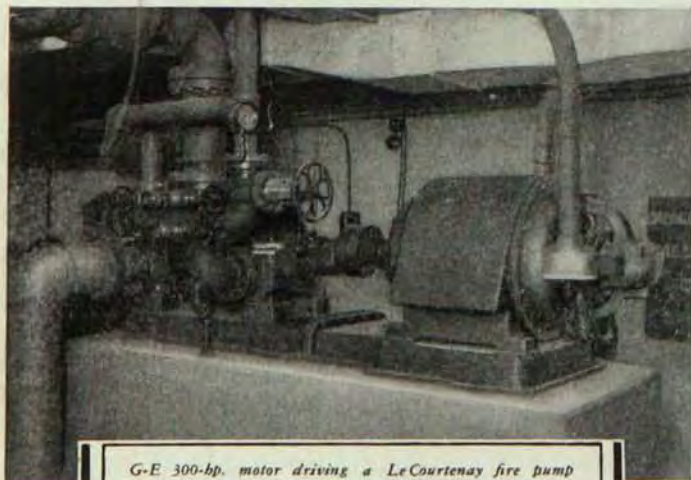
G-E 300-hp. motor driving a LeCourtenay fire pump located in the basement of the Chrysler building, New York City
