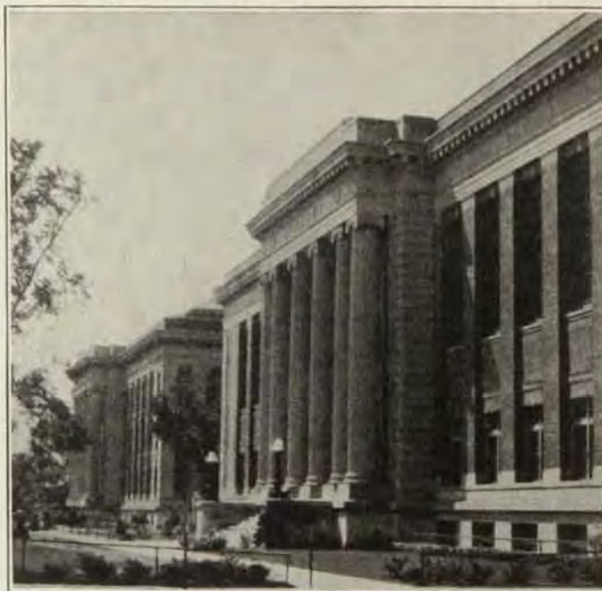
The majestic facades of the Library and the Chemistry Building flank the western edge of the Mall
