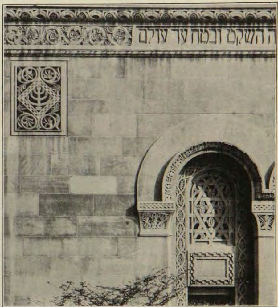
Detail, Temple Emanu-El, New York City. Kohn, Butler & Stein, Architects. Mayers, Murray & Phillip, Associates. Cauldwell Wingate Company, Builders.
