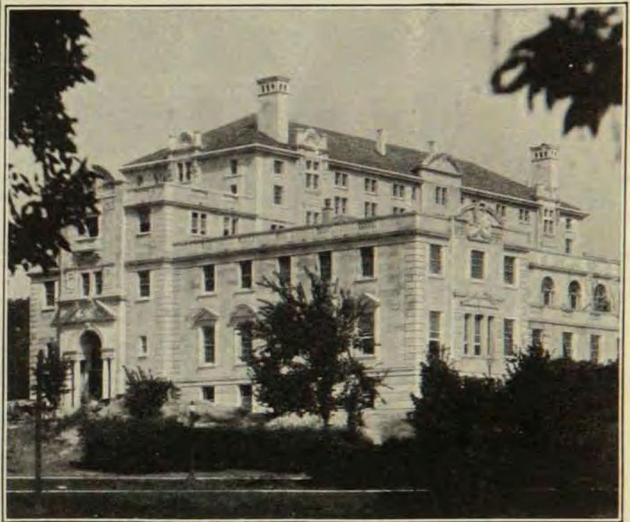
Memorial Union Building, Ames, Iowa. Proudfoot-Rawson-Souers, Architects. Built of Indiana Limestone. A. H. Newmann Company, Builders
