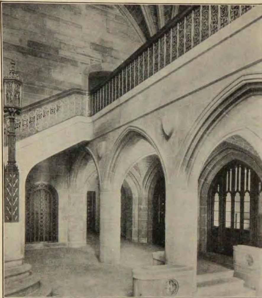
Interior view, Chicago Theological Seminary, Chicago. Riddle & Riddle, Architects. H. B. Barnard, Builder.
