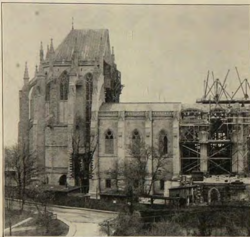
Washington Cathedral in process of construction on Mt. St. Alban, Washington, D. C. Frohman, Robb & Little, architects for the construction of the cathedral, successors to the late Henry Vaughn, the original designer. Indiana Limestone from the quarries of Indiana Limestone Company is being used for this project.
