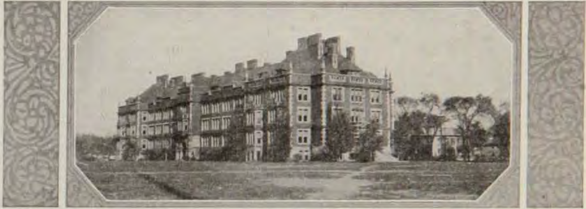
Still one of the campus' most beautiful buildings is Folwell Hall, probably used more than any other campus building.
