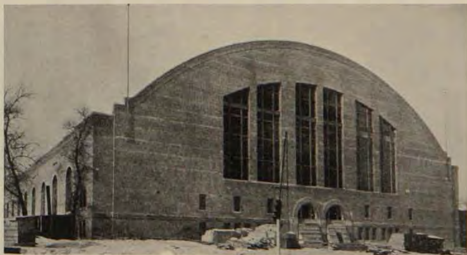
Two days before the dedication game on February 4, the Field House looked like this. This Oak Street entrance end view gives a graphic picture of the tremendous size of the building. The piles of lumber and rubbish are now being cleared away.
