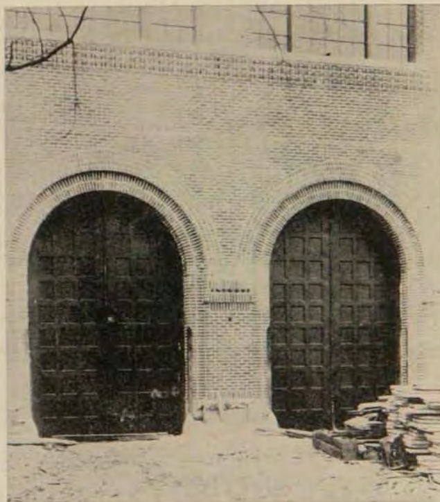
A view of the enormous fireproof doors in the new Field House is shown above. Note how artistic these doors are and how they harmonize with the building itself.
