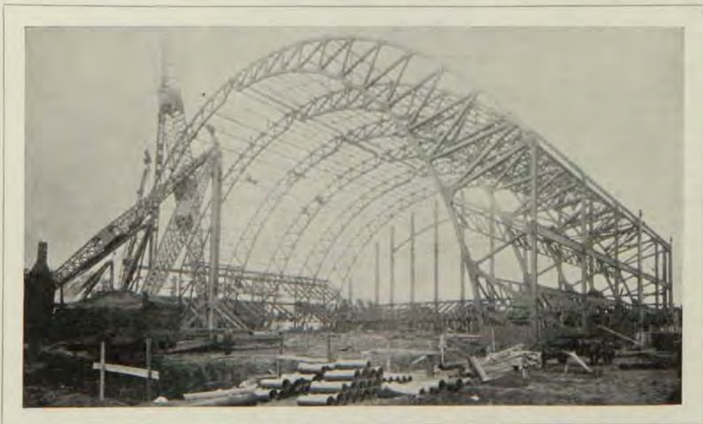
An early construction photograph gives one an idea of the size of the steel girders. Three special type cranes were necessary to erect the girders and were shipped here from the east. This building is the largest ever erected in the northwest.
