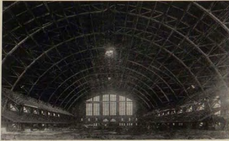
The construction of the steel girders and the suspension of the balconies is unique with the University Field House. The interior steel work is being painted with a light olive green paint to properly reflect the lights without glare to the eyes of spectators.
