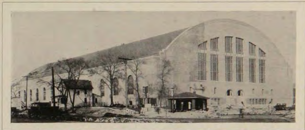
The new University of Minnesota Field House occupies an entire block. The gasoline filling station and the house now being moved away give an idea of the enormous size of the structure which is as high as a nine story building. The building will be surrounded with lawn this summer and will be landscaped.
