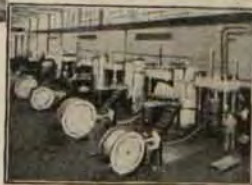
Behind the lines at the great Western Electric cable shop.
