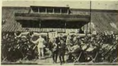
"Here comes '77" was shouted from the stands as the procession approached the stadium. Loud applause followed.
