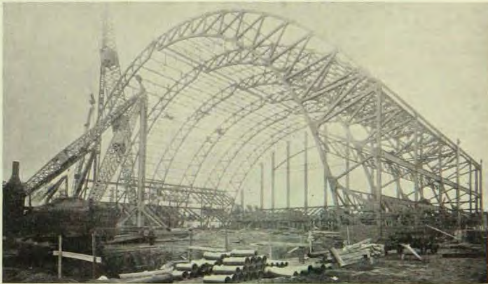
This is how the Field House looked on the morning of September 28, 1927—with fully one-half of the structural steel in place.
