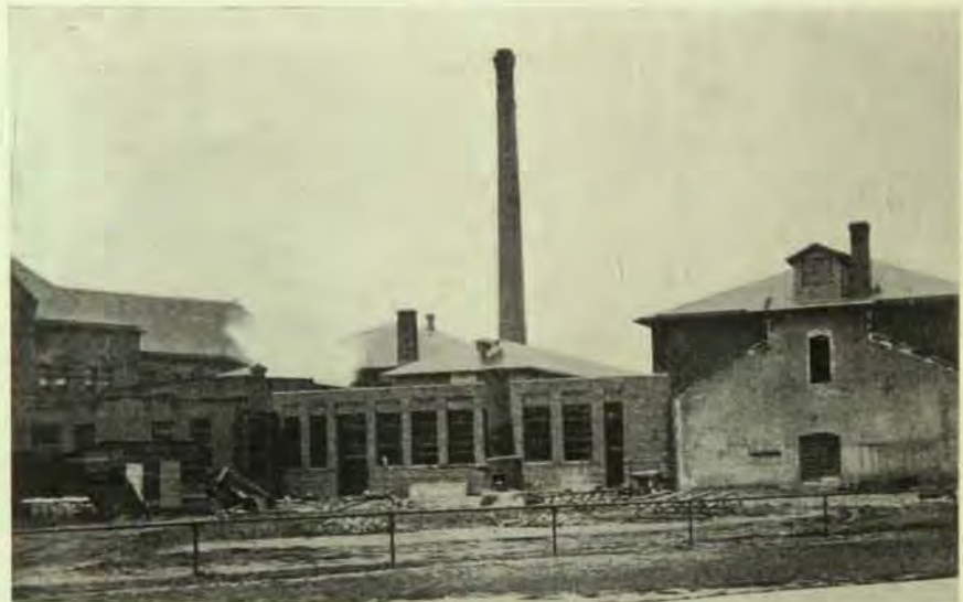
The western section of the Old Mechanical Engineering shop was torn down this fall and a new section added, in order to make way for the Auditorium, soon to be built.
