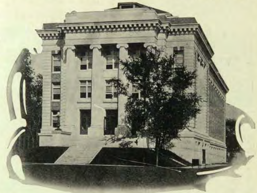
The Administration building, in which are located the alumni office and the editorial and business offices of the ALUMNI WEEKLY, has a new neighbor. The new $450,000 Physics building is now being finished at the right in this picture.
