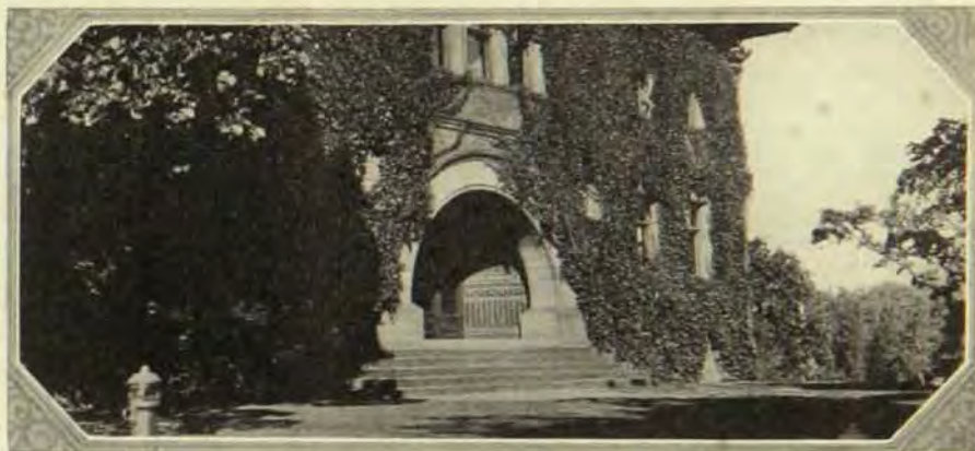
Work on the new Law building is now progressing, auguring a new use for the old law building pictured above.
