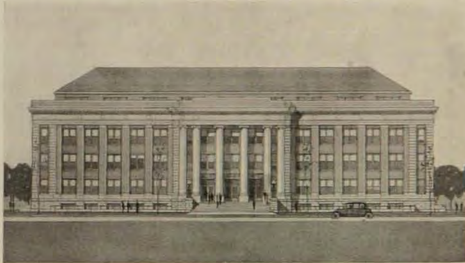
SCIENCE AND RESEARCH TO HAVE NEW BUILDING Work is progressing rapidly on the new $450,000 Physics building located directly opposite the new Library building on the Mall.
