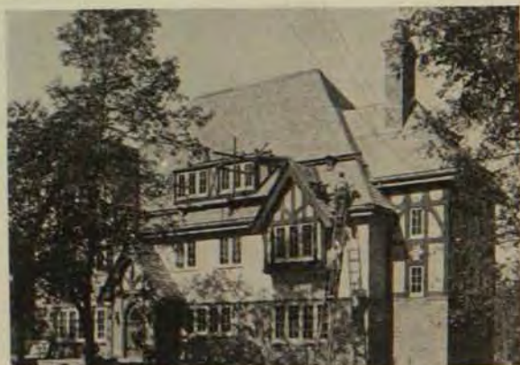
FINISHING ALPHA CHI'S ROOF
