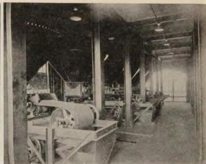
ORE BIN AND FEEDERS
