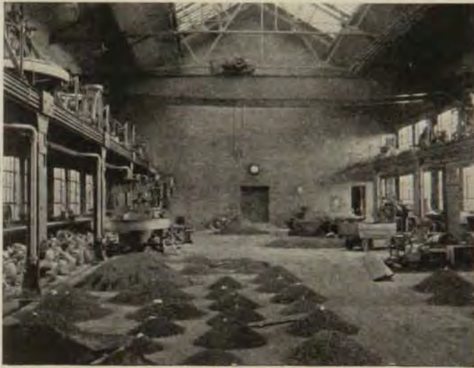
Samples of iron ore under test are carefully labeled and the results recorded. The laboratory is so constructed that apparatus and machinery not in use may be stored under and on the mezzanine floor.
