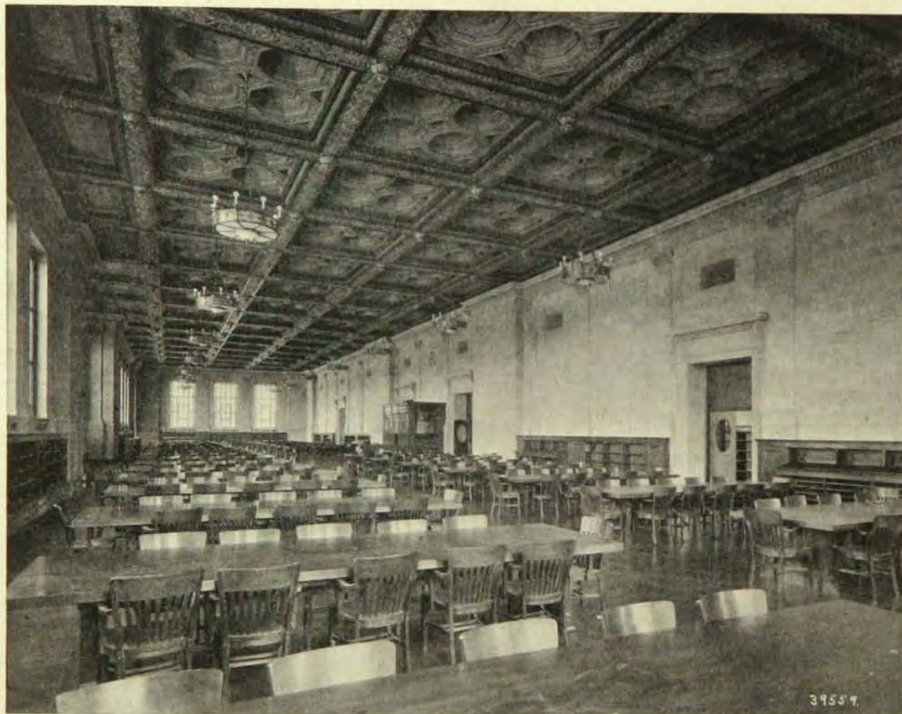
The Main Reading room covers the entire front of the Library. Equipped with long tables, individual chairs and diffused lights, it is one of the best rooms for quietness and study in the University. The table lights, which had not yet been installed when this picture was taken, may be seen on Page 14. The floor is covered with linoleum and the ceiling is done with great elaborateness of design.
