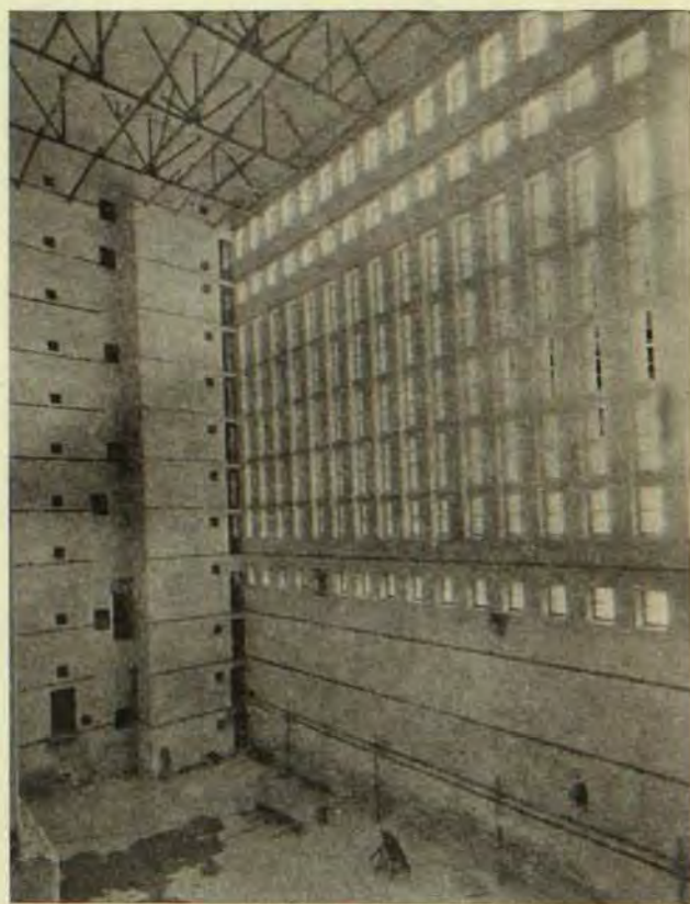
The "well" or stack room as it appeared before the steel stacks were erected. This room now houses twelve stack floors. The upper eight are finished and have a capacity of 750,000 volumes.
