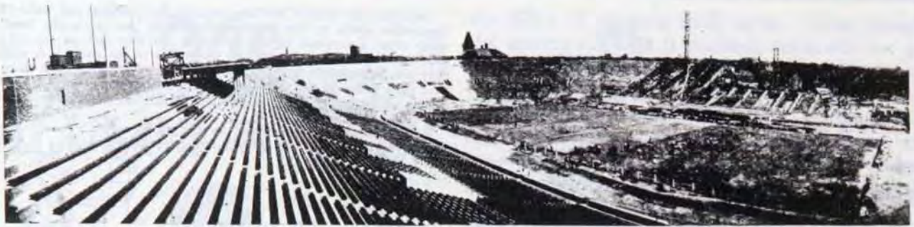
This view gives you a good opportunity to note the rapid progress being made on Minnesota's Memorial Stadium. At this end the entire portion is complete from the redwood seats to the brick surrounding wall. Note the flag poles at the left top, from which flags and streamers will fly to add to the festiveness of the football games. The roof-house at the left is to be glass-enclosed and will house representatives of the press, scouts and official visitors. Photograph taken Friday, July 18.
