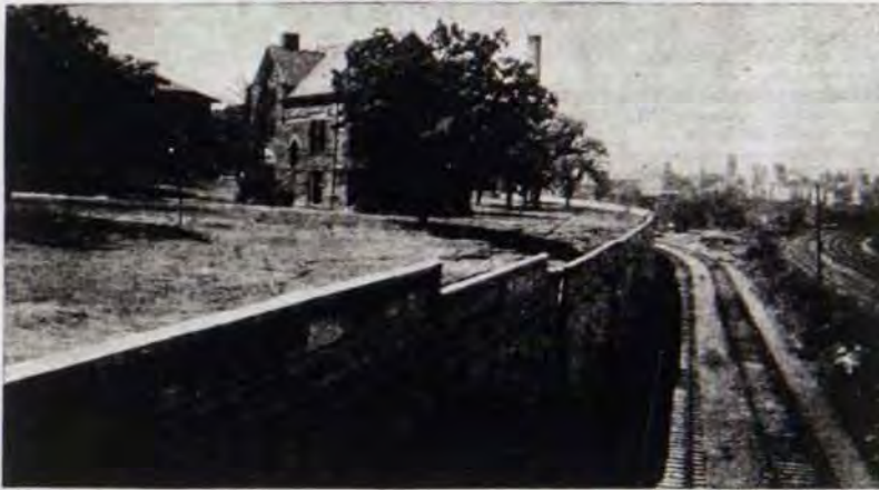
During a cloudburst the early part of June, the loose dirt filled in so heavily against the new retaining wall on the northwest side of the campus that a large portion was caved out about two feet at the top as shown in the picture above. This wall was put in last year when a portion of this side of the campus was cut away to allow the Northern Pacific railway trackage space when the tracks were removed from the center of the campus. The dirt filled in added much lawn space that originally was roughly overgrown with brush. The building in the left background is the Publications building (formerly the Students' Christian association and then the Music building). The overturned skyline of Minneapolis is dimly discernable in the distance.
