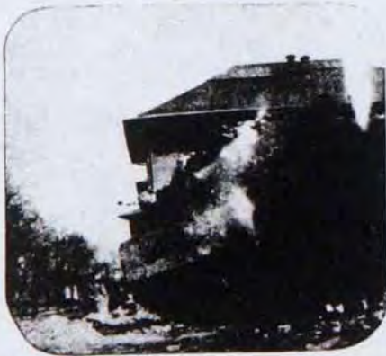
Many changes have been made on the campus the last two years. The old must give way to the new in this day of progress. Here, the wrecking of the old storehouse, (former medical building) is in progress.
