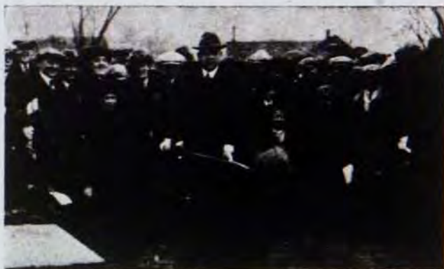
President L. D. Coffman turns the first dirt in the erection of Minnesota's new memorial stadium. (Photo by U. of M. News Service)
