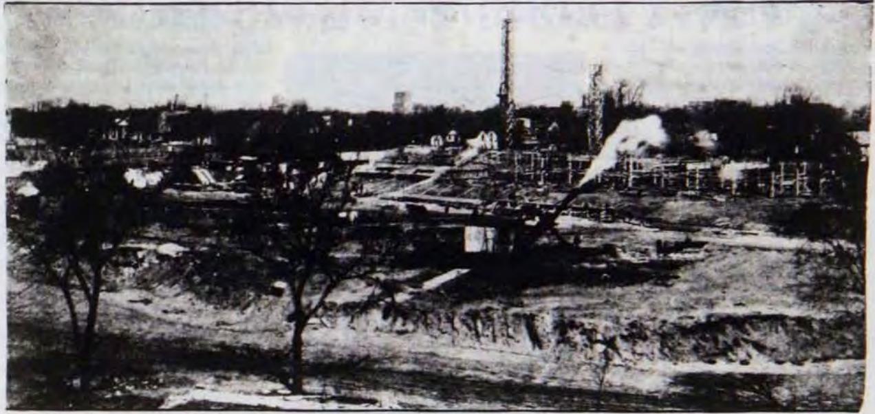
How fast work on the Memorial Stadium is progressing is shown in this picture taken April 18. The steam shovel in the foreground is loading dirt into the dummy railway cars and is used to fill in the Northern Pacific tracks cut which has been vacated. Two concrete towers in the distance are set on "rollers" and will be moved about the structure as each section is poured.
