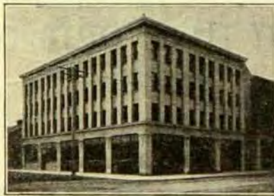
OCCUPYING THE ENTIRE BUILDING
