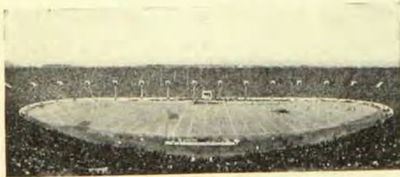
The Yale bowl, one of the first stadia of this kind ever constructed. The Minnesota stadium will be built in the form of a bowl and is so designed that a second section may be added later
