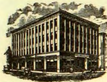
OCCUPYING THE ENTIRE BUILDING
