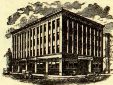
OCCUPYING THE ENTIRE BUILDING
