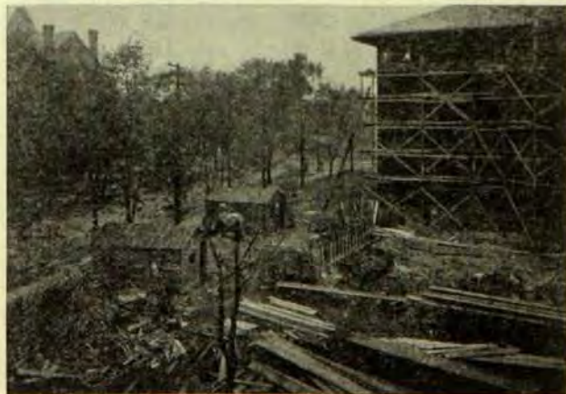
The Union addition getting under way.
