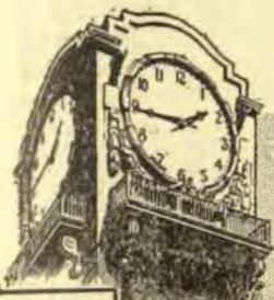
Tower clock wound automatically by one-half horse power motor.
