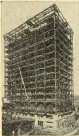
Structural Steel For All Kinds of Buildings.
