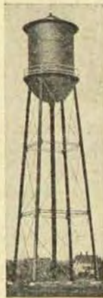
Water Tanks, Towers and Stand Pipes.
