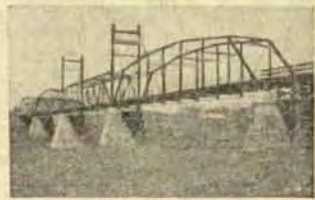
Highway and Railroad Bridges.
