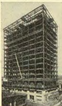
Structural Steel For All Kinds of Buildings.
