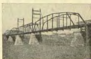
Highway and Railroad Bridges.
