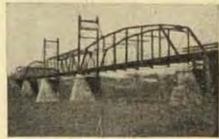
Highway and Railroad Bridges.
