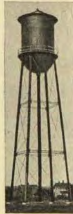
Water Tanks, Towers and Stand Pipes.
