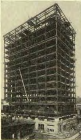
Structural Steel For All Kinds of Buildings.
