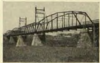
Highway and Railroad Bridges.
