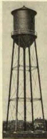
Water Tanks, Towers and Stand Pipes.
