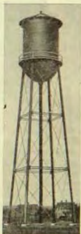
Water Tanks, Towers and Stand Pipes.
