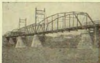
Highway and Railroad Bridges.
