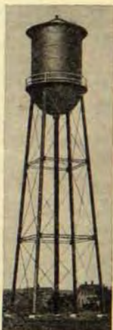
Water Tanks, Towers and Stand Pipes.
