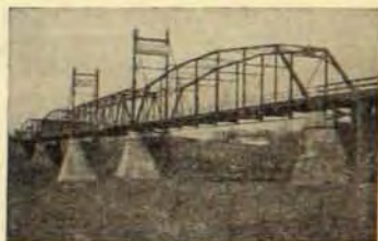
Highway and Railroad Bridges.
