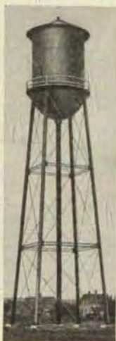
Water Tanks, Towers and Stand Pipes.
