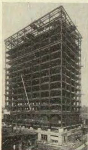
Structural Steel For All Kinds of Buildings.
