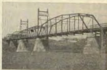
Highway and Railroad Bridges.
