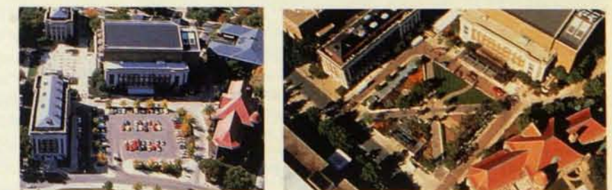
Before and after: The grounds crew maintains the plaza garden above the Church Street Garage. The land used to be a parking lot.
