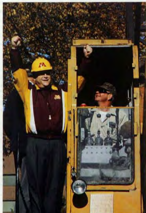
President Yudof took the first swing with the wrecking ball to take down the East River Road Ramp.
