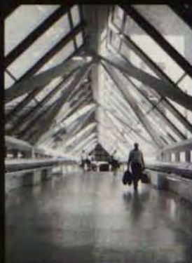
Minneapolis/St. Paul International Airport, Skyways and Vertical Circulation Tower
