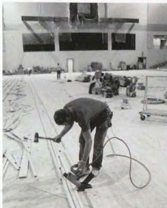
The hardwood floor was installed the week of October 4, 1993
