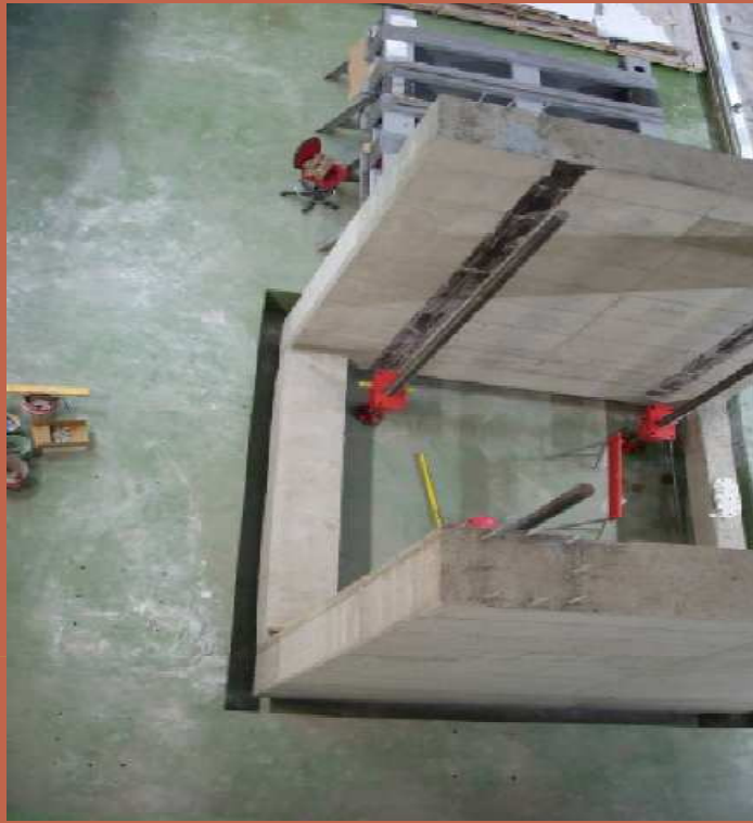
Hut construction: April 2008 status
