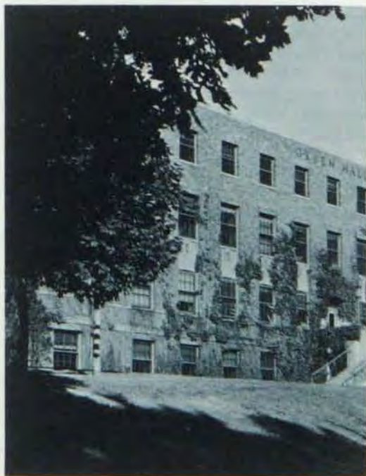
GREEN HALL, which houses the School of Forestry on the St. Paul campus, needs to be remodeled for additional research program space.
