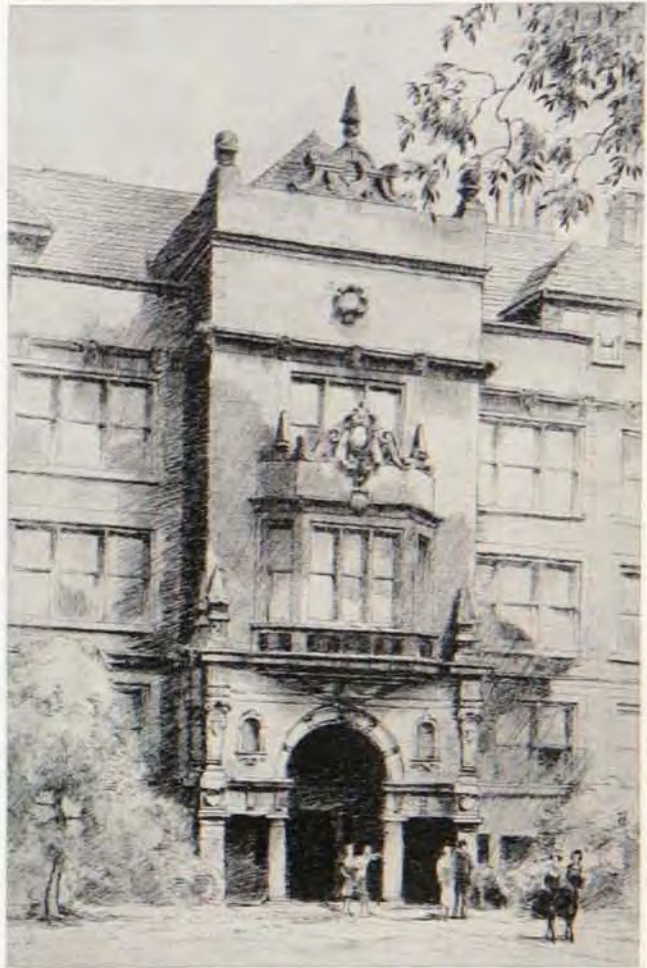
FOLWELL HALL, WHOSE CONSTRUCTION WAS BEGUN IN
