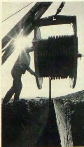
One of our newest routes is a blast-resistant cable that can handle over 9000 multi-channel conversations.
