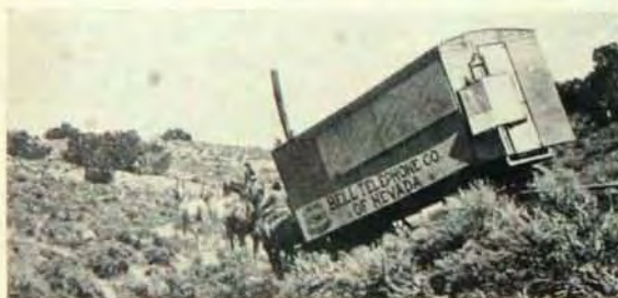
Installers of the first transcontinental line had to surmount hardships of windstorm, ice and scorching heat combined with rugged country.
