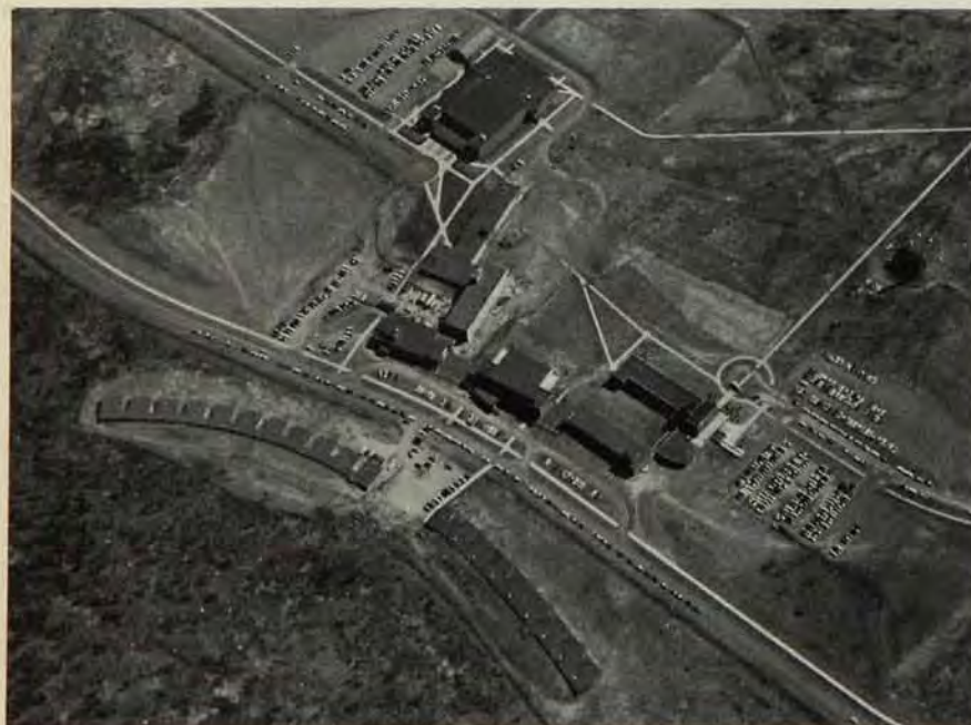
The new Duluth campus area has two sets of student housing, one in use and the other to be ready by the fall of 1959. In use is the residence hall (right, foreground) which accommodates 64. Under construction is a similarly-shaped oblong building (left, foreground).
