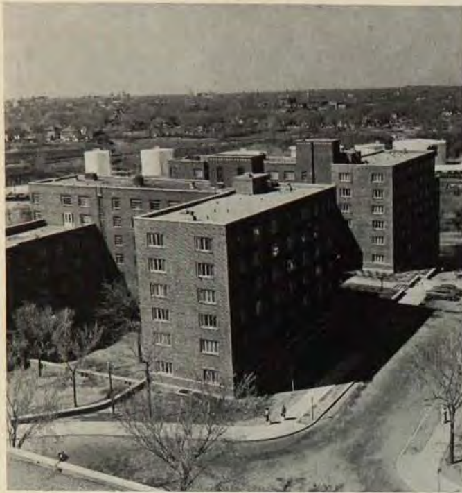
The new wing of Comstock Hall (right foreground) is the same as the older wing (left background.)
